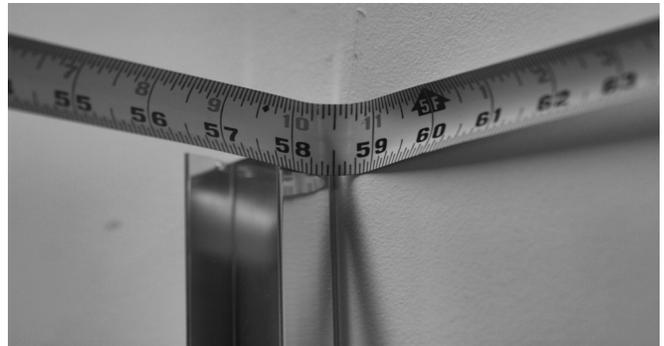
Step 19: Locate the Header and accurately mark the Header where you are about to cut. Place the Header in the miter box and line up the mark on the header against the straight slot, using a Hack Saw cut the header to length.
