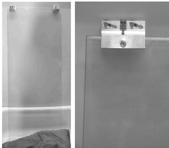
Step 24: The outer glass panel should be located on the opposite Side Jamb of the Shower Head. Make sure you have good contact with the 3 bumpers. If they do not all make good contact with the glass, then remove the outer panel from the header and adjust the rollers to make good contact. **MAKE SURE THAT THE ROLLER SCREWS ARE TIGHT.** Reinstall the panel as in Step 23
